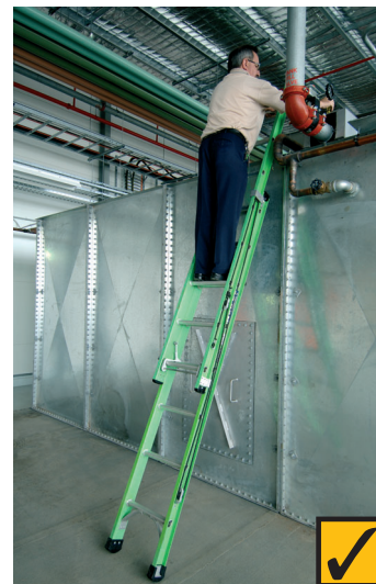
4.0 Person using a ladder working near the edge of a small structure – this situation is okay where the task is light and of short duration and the person can face the ladder and not over-reach.
